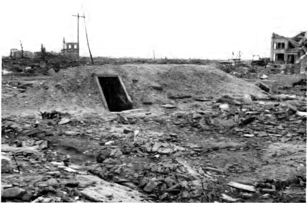
Photo No. 17. HIROSHIMA. Typical, part below ground, earth-covered, timber framed shelter 300 yds. from the centre of damage, which is to the right. In common with similar but fully sunk shelters, none appeared to have been structurally damaged by the blast. Exposed woodwork was liable to "flashburn." Internal blast probably threw the occupants about, and gamma rays may have caused casualties. See paragraph 40.
